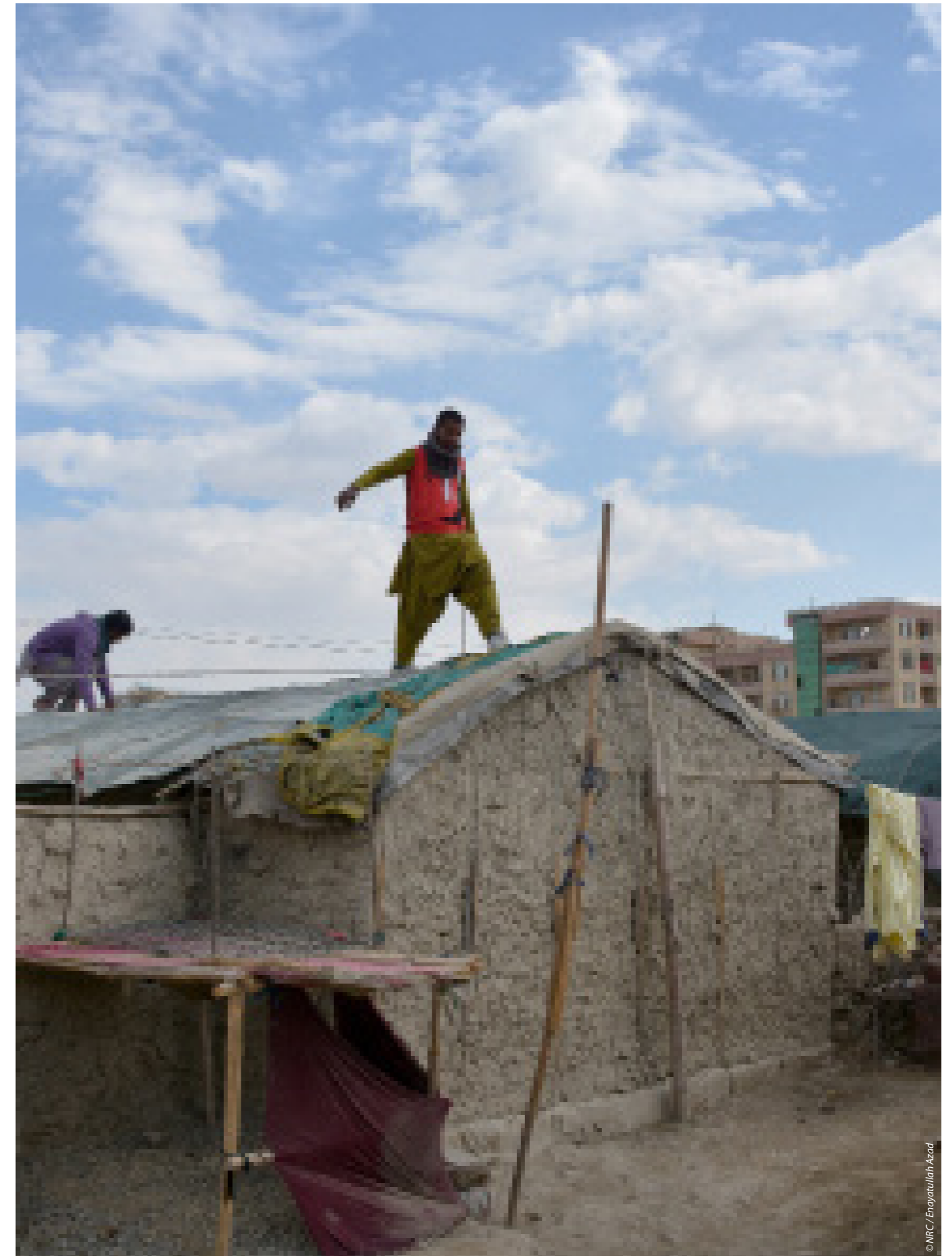
Mud brick and tarpaulin shelter in the Hewadwal IDP settlement in east Kabul.
