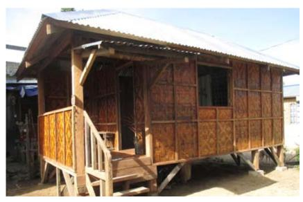
In August 2015, CRS piloted the use of coco lumber panels for walling in the direct-build shelters to respond to community feedback on the use of *amakan* bamboo walling. Beneficiaries felt the *amakan* bamboo walling was of a poor quality, could be seen through at night and let the rain in. The use of the coco lumber panels did not increase the price of the direct build.
