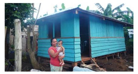
In December 2014, CRS changed the roof on the Pablo direct-build shelters from a gabled roof to a hipped roof.
