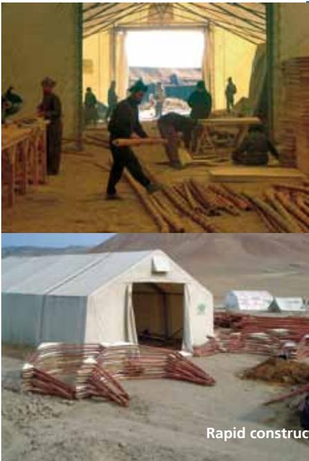
Rapid construction process - materials were prefabricated in a warehouse and assembled on site
