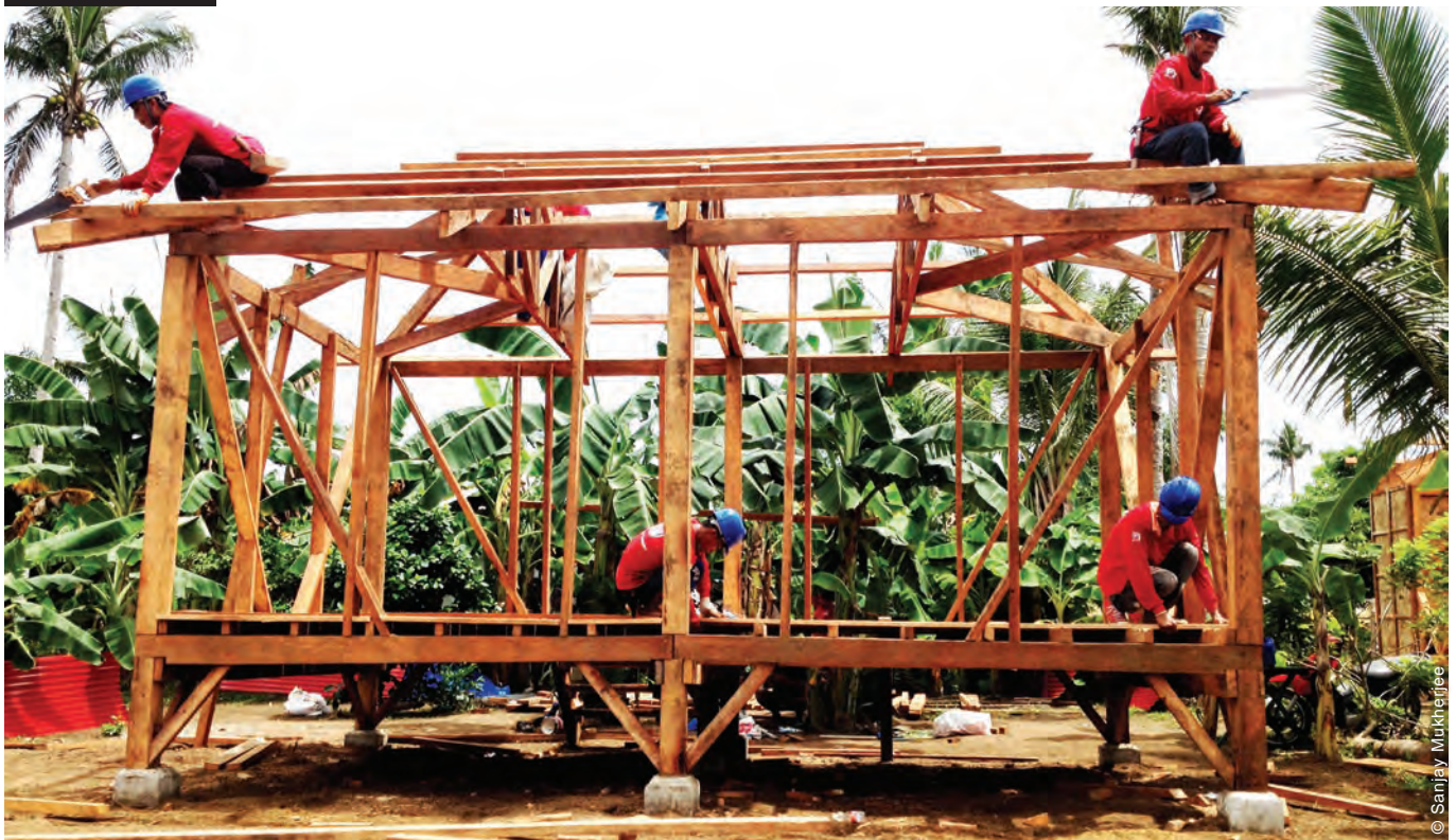
Core shelters were built in several batches by construction teams that included the beneficiaries. Material supply and monitoring were managed by the organization.
