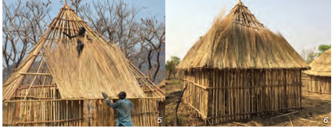
Skilled workers were paid to build shelters in the following stages: 1. The site was demarcated and structural poles were erected. 2. The structure and door were built. 3. Wall matting was added. 4. The roof structure was built. 5. The roof was thatched. 6. Once the thatching was complete, the Tukul was ready to be plastered with mud (see picture on the opposite page).
