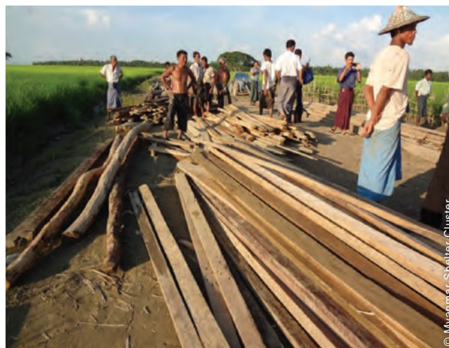
© Myanmar Shelter Cluster Construction materials were supplied by the government to rebuild the houses of IDPs affected by the violence (Thi Kyar IDP Camp, Mrauk-U Township).
