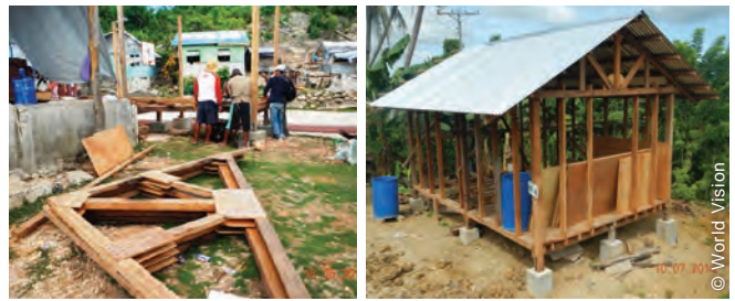
The project prefabricated trusses and built transitional shelters.
