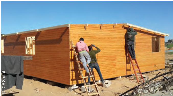
Timber-frame buildings were built on a platform with a plywood floor. From left to right, top: 1. Laying the foundation and ground beams for the transitional shelter. 2. Installing plywood layer over the ground beams. Bottom: 3. Fixing the external wall cladding with screws. 4. Contractor staff placing CGI roofing on the shelter.
