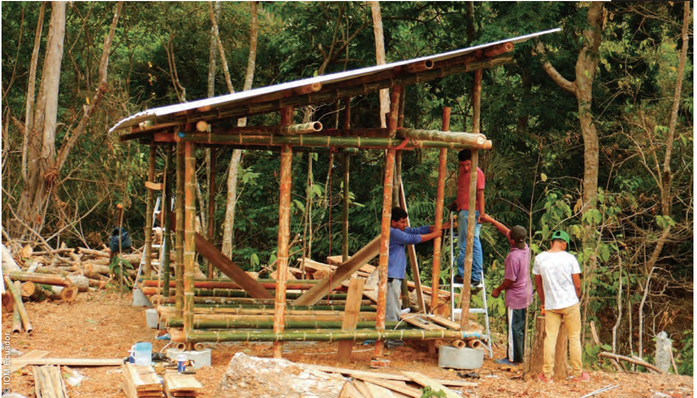
Although initially challenged by the government, many agencies proposed temporary or transitional shelter solutions, that would use local materials (such as bamboo) and provide adequate living conditions in the time span between the emergency phase and the formal reconstruction process (planned by the government).
