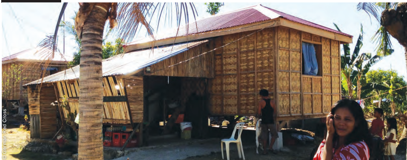
Multiple programme options were encouraged in response to Typhoon Haiyan, one of them being the construction of transitional or core shelters.
