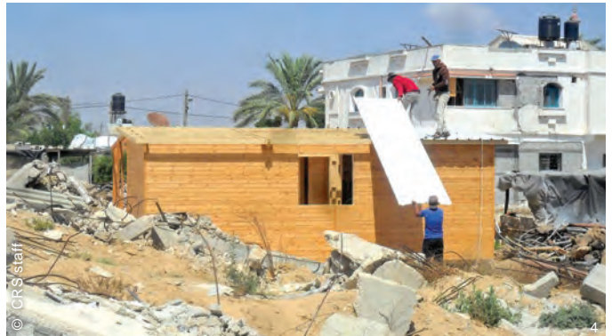
Timber-frame buildings were built on a platform with a plywood floor. From left to right, top: 1. Laying the foundation and ground beams for the transitional shelter. 2. Installing plywood layer over the ground beams. Bottom: 3. Fixing the external wall cladding with screws. 4. Contractor staff placing CGI roofing on the shelter.
