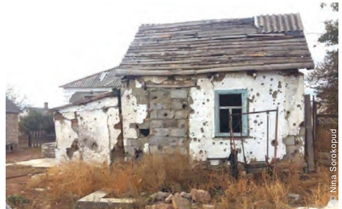
Multistorey buildings (top) and houses (bottom) in conflict zones sustained significant damage due to shrapnel punctures, and required urgent repairs.
