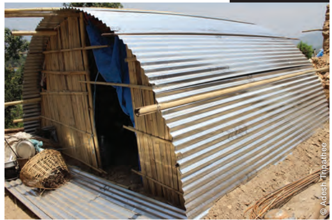
Some people used the materials provided to build temporary shelters according to the organization's design.
