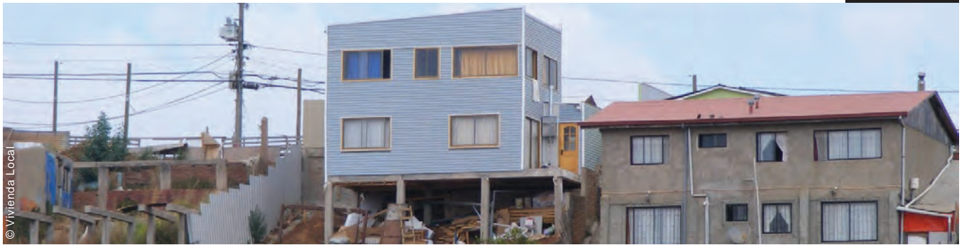
Architects and local NGOs helped affected people rebuild their damaged houses, thanks to the “assisted self-construction” subsidies provided by the government.
