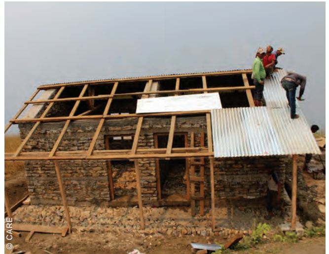
Houses were repaired also using the materials provided by humanitarian organizations, such as CGI sheets and timber.
