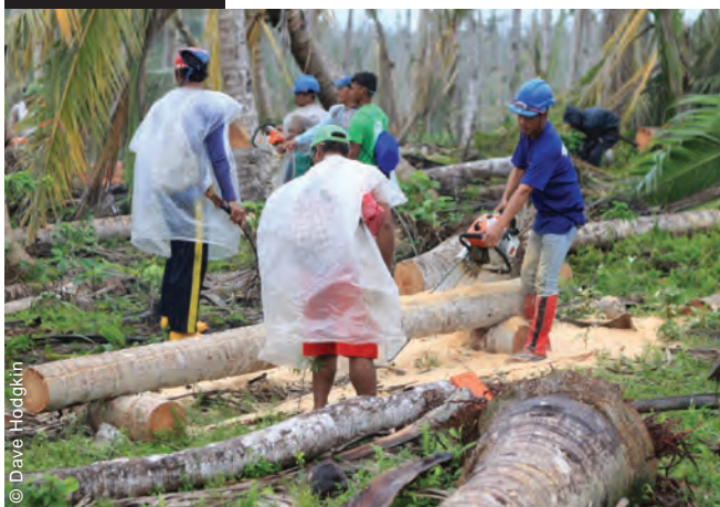
The project used a flexible approach to reuse fallen coconut trees to set up a large-scale shelter response. Most of the milling was done by licensed chainsaw operators, directly where the coco-lumber was sourced.
