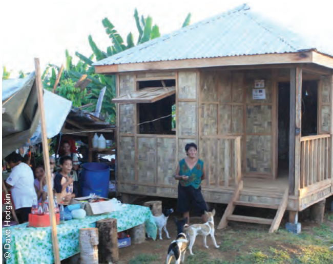
Transitional shelters were used as a basis to recover. Families would personalize the shelters and add small stores and other temporary structures outside the shelters, which served as places for livelihood activities.
