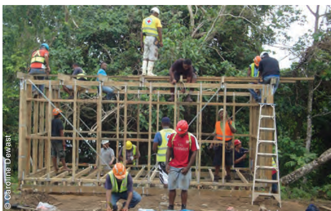
The Shelter Cluster Fiji conducted Build Back Safer training of trainers.
