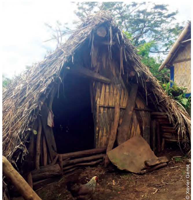
Most of the housing in Vanuatu was built according to vernacular techniques.
