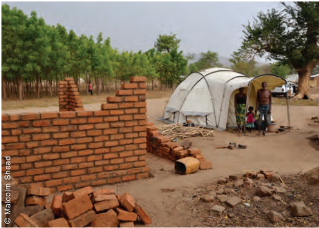
By pitching the tent on their home site, people were able to start to rebuild their damaged houses. Supporting return was essential for enabling early recovery.
