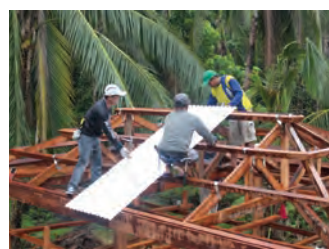
The project used locally available materials (e.g. the amakan sheet, left) and safe construction techniques, including bracing, strong trusses and roof strapping.
