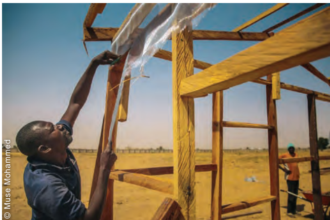
Shelters included specific details, such as mosquito nets in the open gap beneath the roof, which was intended for ventilation.
