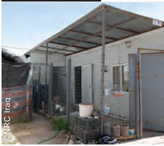
The project worked on a variety of upgrades focused on improving the accessibility and Quality of Life of individuals with disabilities. From left to right: Shaded area and fencing around prefab shelter. Concrete slab improving wheelchair access. Fold out support railing. Shaded entrance and support posts for better access.
