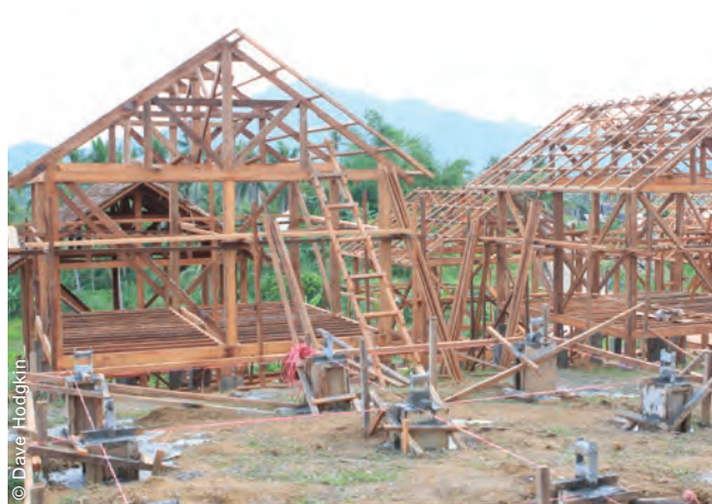
In a few cases, transitional shelters were built in resettlement sites, such as this one in Tacloban, rather than on people's original plots.
