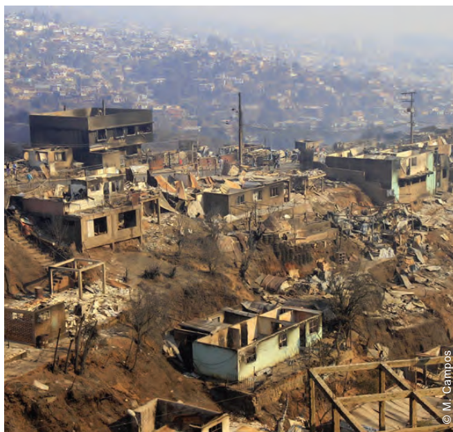
The damage caused by fires in the ravines of Valparaíso is often extensive. Entire neighbourhoods were burnt down by the fire in April 2014. The same areas were again affected by a fire in January 2017.
