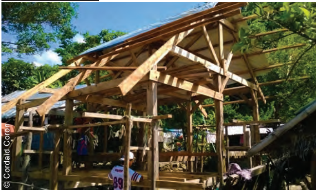
Shelters were constructed as a way to build community resilience.
