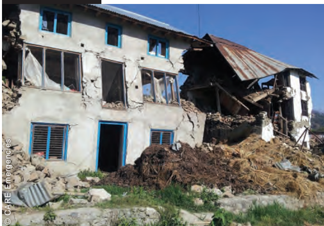
© CARE Emergencies Many constructions affected by the earthquake were masonry buildings. The project provided materials to make urgent repairs to damaged homes, or build temporary shelters.
