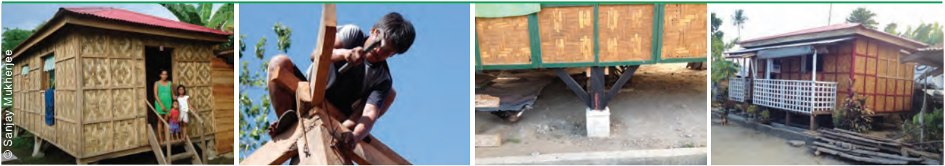
Safer building practices were promoted, such as strapping of roof structures, bracing and proper detailing of the foundations (raised and made of reinforced concrete).
