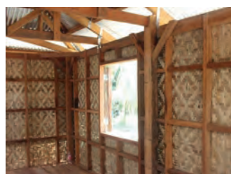
The project used locally available materials (e.g. the amakan sheet, left) and safe construction techniques, including bracing, strong trusses and roof strapping.
