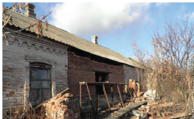
Interventions included housing repairs (Starohnativka, Dec 2015).
