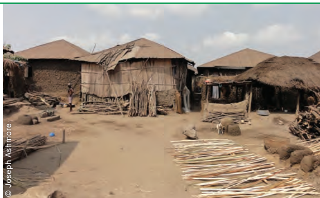
Shelter repair kits and cash grants were provided to support return to areas of origin after the floods.
