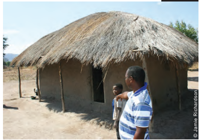
Many of the traditional houses withstood the floods, as they were built with contextually appropriate features, such as roof overhangs and raised platforms.
