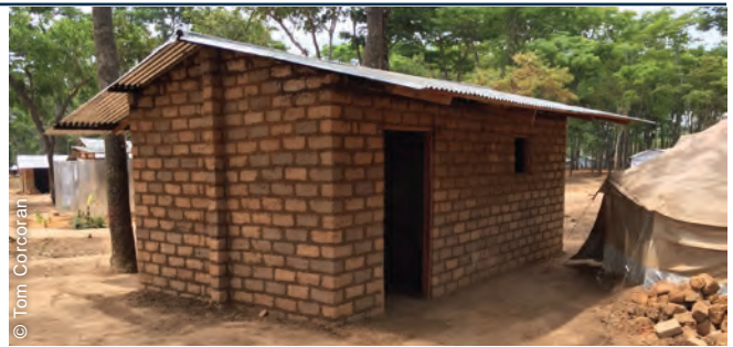
Lime-stabilized transitional shelters were built in Nduta refugee camp. The emergency shelter solution (tent), where the family was living during the construction, can be seen on the same plot near the shelter.
