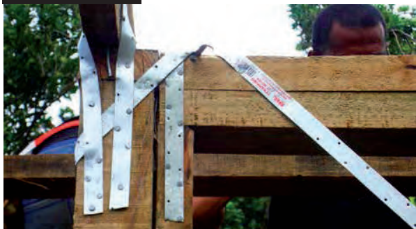
Strapping should be long enough to hold four (4) nails on each side. Note that the diagonal bracing is stretched tight and is wrapped around the frame at the ends. Note also the double top-plate to support the roof frame.
