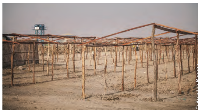
Shelter frames were built by contractors.
