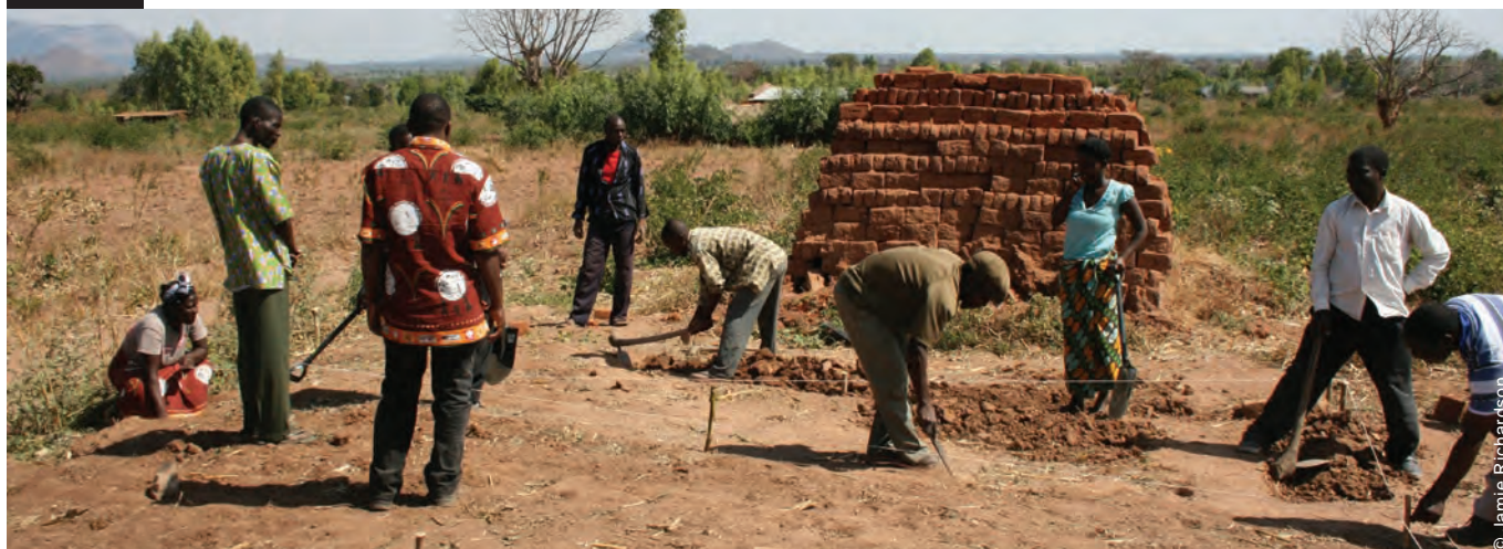
People were given technical trainings and built model houses as part of the project. Here they are working on setting out the foundations of a model house..
