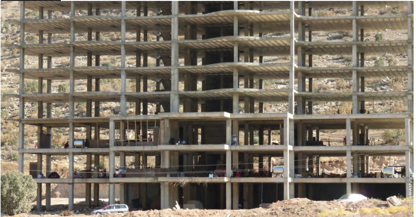
Unfinished buildings were occupied by some people. Where agreements were possible with landowners, repairs, light or durable upgrades were made. In some cases, frame tents or sealing-off kits were provided.
