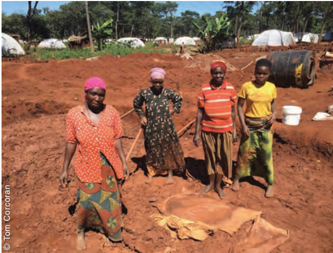
Women were involved in mixing clay, lime and sand (Nduta camp pilot project).
