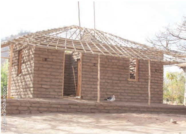
Model homes were built, according to traditional designs. Additionally, materials were provided and cash-for-work grants for the 10% most vulnerable households.
