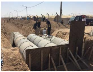
One site was vulnerable to heavy rains and suffered minor flooding during winter. In 2018, storm-water drainage channels and culverts were upgraded.
