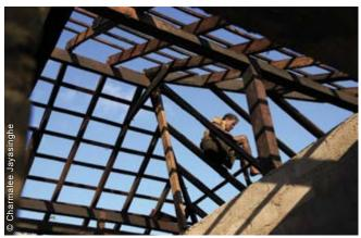
Roof work in progress in Vavuniya district. DRR features were included in roofs, foundations and walls. The gradient was increased to enable better run-off.
