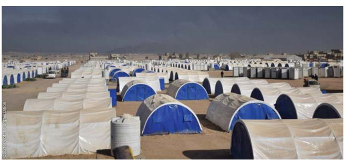
Government standard tents of 6x4m were installed in clustered blocks of 20 each. Space for extensions was minimal but, after families had moved in, upgrades were conducted to the floor and electricity was installed. Partners could then build service facilities in specific blocks pre-allocated in the site plan.
