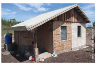
The project provided core houses with light-weight extensions, based on a common rural design. The houses included a gutter and a water tank for rainwater collection
