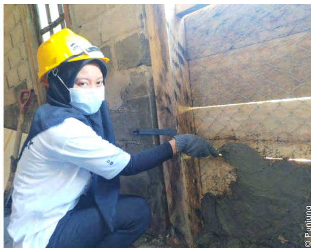
Construction training using retrofitting method (ferrocement) for women in Karampuang Village.
