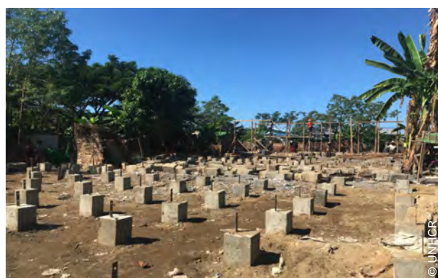
The reconstruction work incorporated pre-cast footings for extending the lifespan of the timber frames, while improving the anchorage of the building to the ground.
