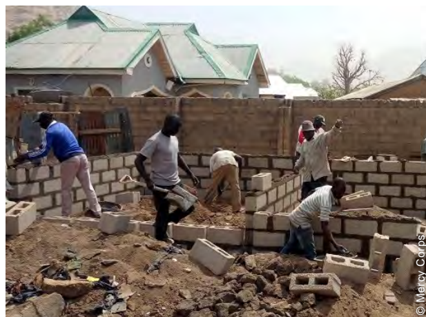
Construction of the permanent shelters using blockwork.
