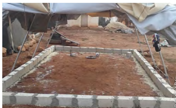
Tent leveling construction activities - (above) Building of the tent base perimeter with mortar blocks, November 2021. (below) Filling of the tent base with aggregate before the final cement layer, November 2021.
